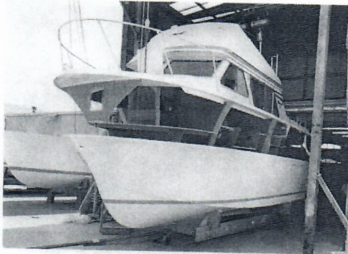
The deck and liner are lowered onto the hull.
